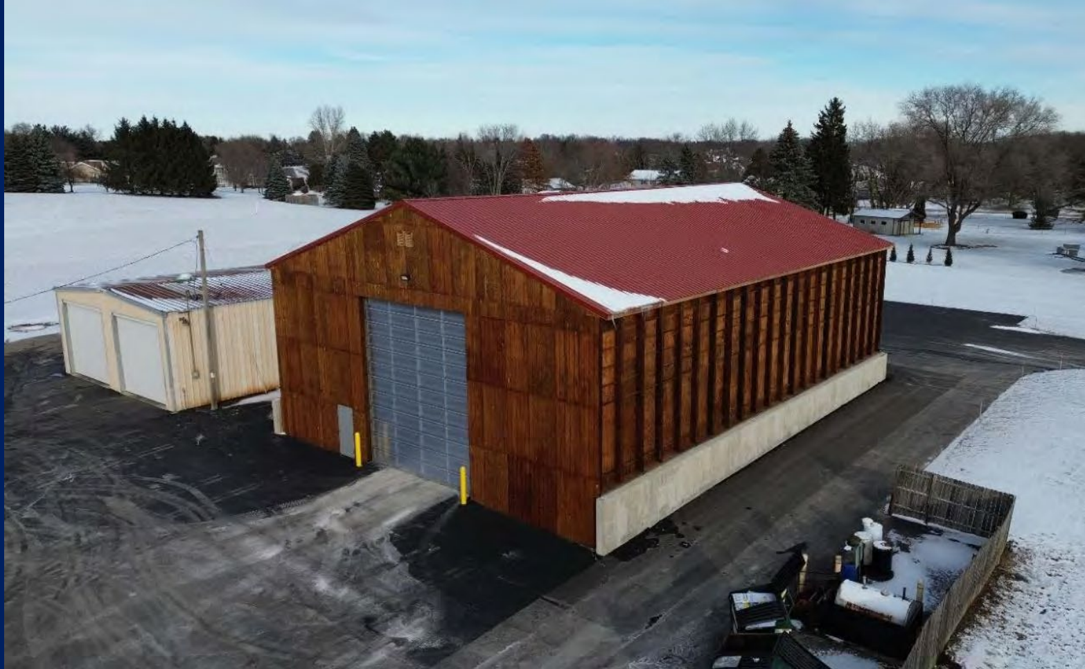
Salt Storage Facility - Example
