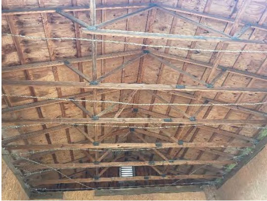
Photo 19 – Broken Truss
