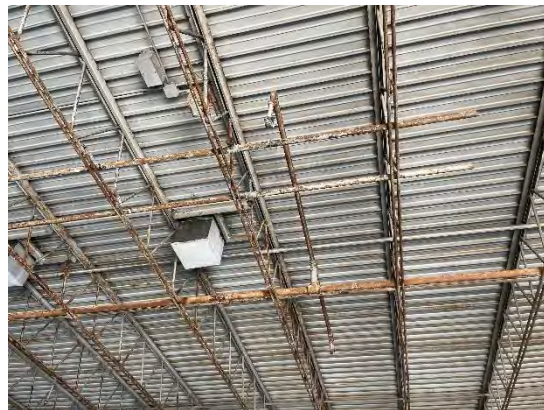
Photo 4 – Corroding Metal
