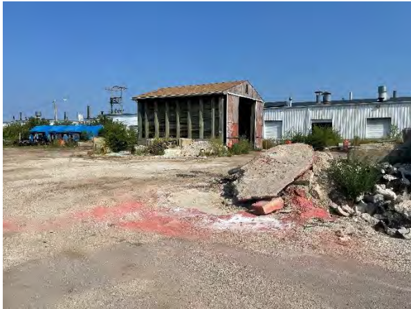
Photo 3 – Topsoil Storage Building
