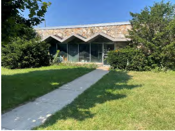
Photo 1 - Building Exterior – East Side
