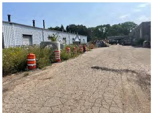
Photo 6 – Asphalt Cracking
