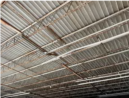
Photo 3 – Corroding Metal
