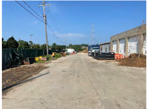
Photo 4 – Southern Concrete Drive – Facing West
