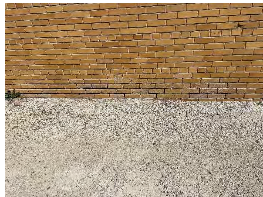
Photo 12 – Deteriorating Mortar
