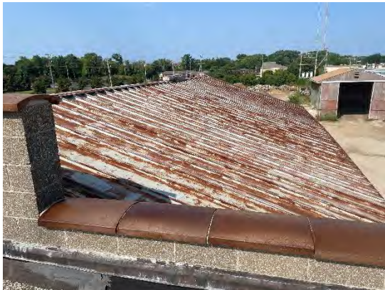
Photo 3 – Sloped Corrugated Metal Roof
