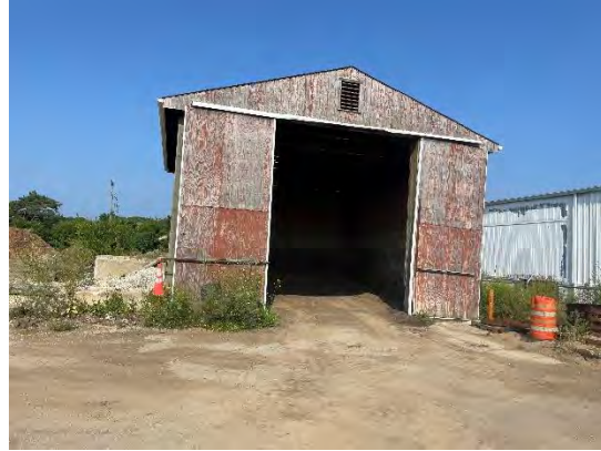
Photo 24 – Faded Paint
