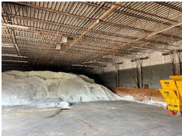
Photo 5 – Building Interior – Salt Storage
