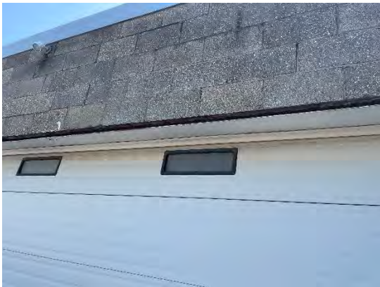
Photo 21 – Damaged Lintel
