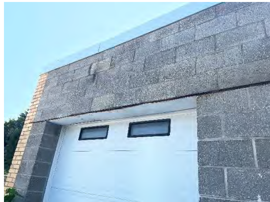
Photo 22 – Damaged Lintel
