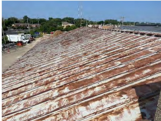
Photo 4 – Sloped Corrugated Metal Roof
