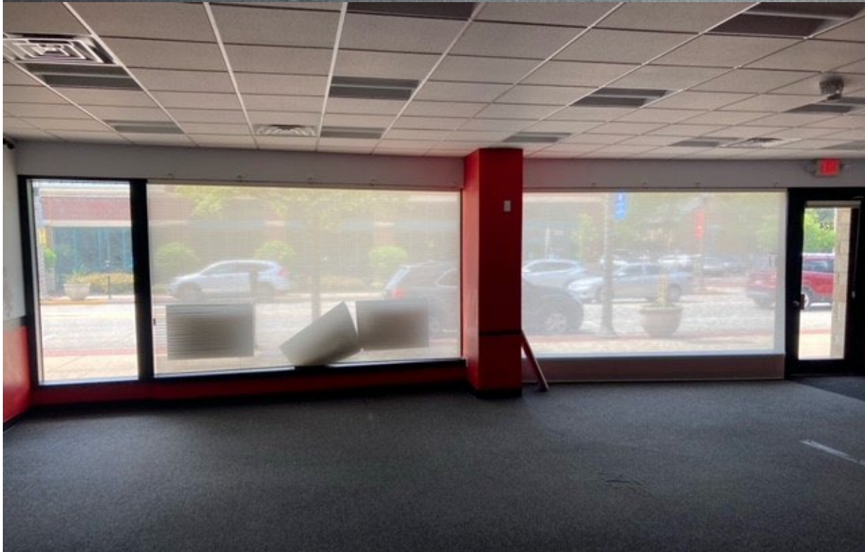
Phase 2B – interior former 9 Round
