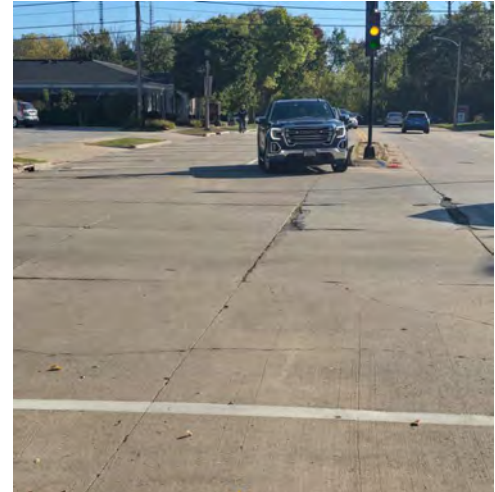
1. Opposing left-turning truck obstructs driver's view of oncoming through traffic, illustrating visibility challenges caused by negative offset.
