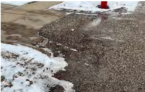
Asphalt Overlay Driveway
