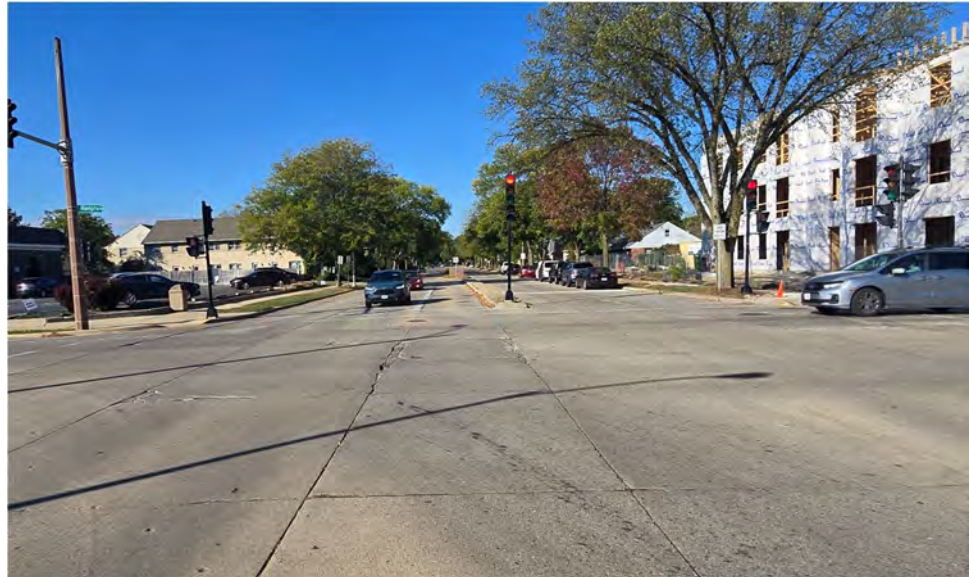
2. Limited signal visibility for northbound movements due to post-mounted heads and lack of overhead indications
