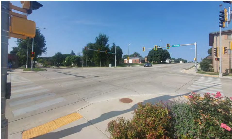
New traffic signal equipment, improved signal timings, updated pedestrian facilities, and high visibility block-style crosswalks were just a few of the improvements.
