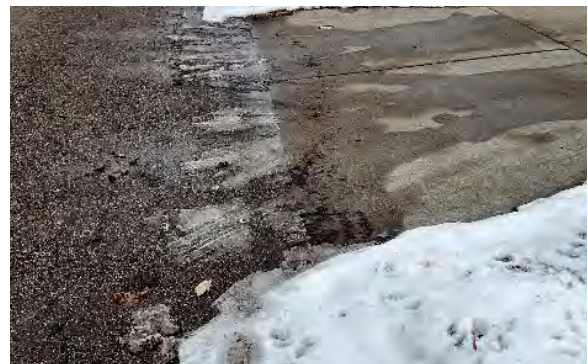
Asphalt Matching New Driveway Approach
