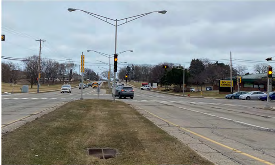
Before the HSIP project, there was negative offset for left-turn movements, poor signal head visibility, and substandard pedestrian accommodations.
